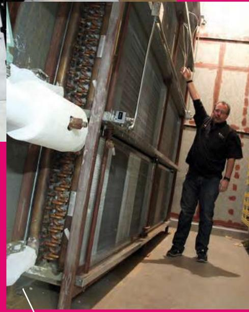
*Building Operator Jason Nieskens stands beside the new cooling coil installed in the Arts Commons air circulation system. © Alex Bonyun*
